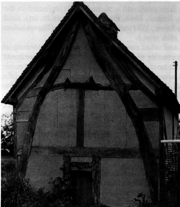
Fig. 4 Hill Croome, Upton-upon-Severn, Hereford and Worcester. The only known cruck-trussed dovecot Avoncroft Museum of Buildings
